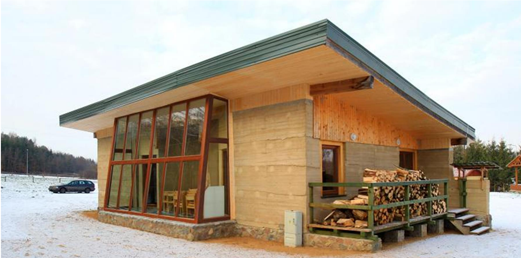
Experimental building of the Warsaw University of Technology with rammed earth
